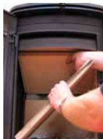
3. Tip the other side brick and remove it from the fire chamber.
